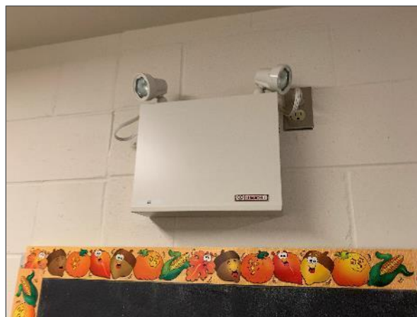
Lead-containing batteries in emergency lighting.
