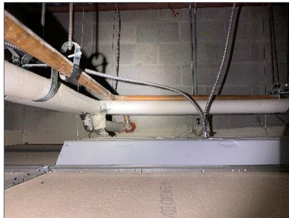
Pipes insulated with non-asbestos fibreglass.
