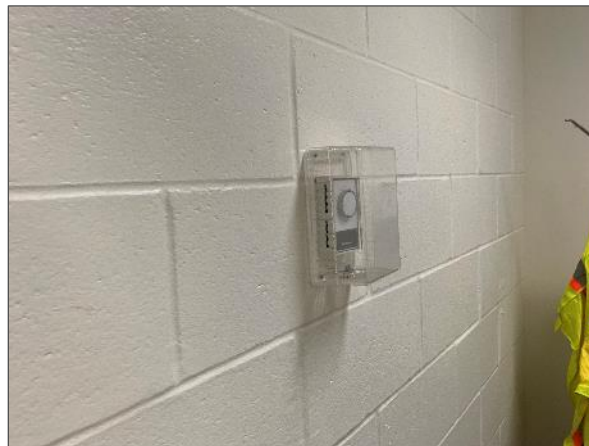
Thermostat containing liquid mercury ampules.
